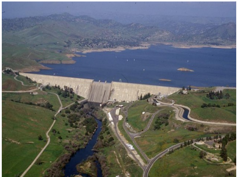
Millerton Lake Dam
