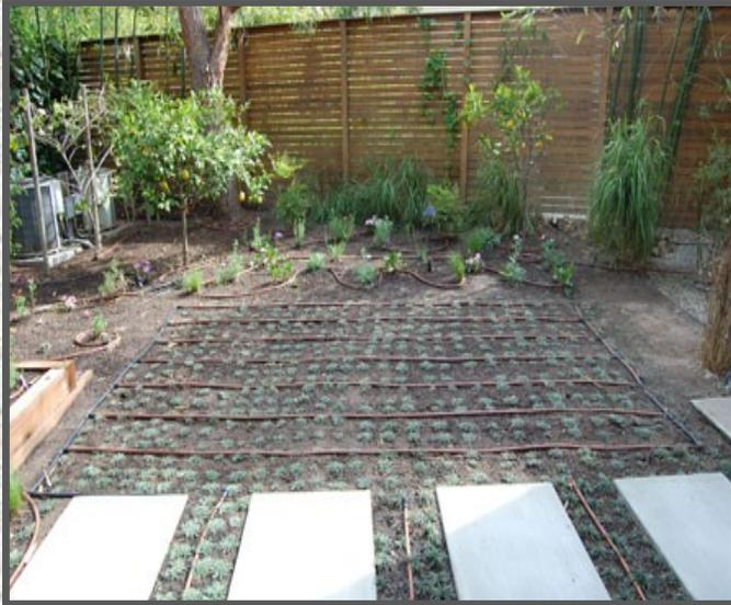
***Drip irrigation using in-line 1/2" tubing***
